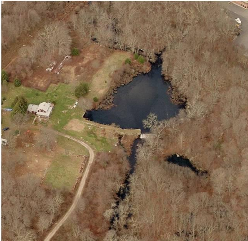
Aerial photo of dam #2 off of Lane Way, Stonington
