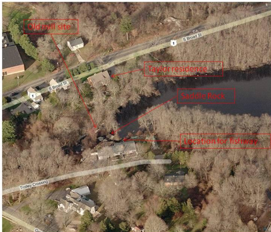
Aerial photo of dam #1 off of South Broad Street, Stonington
